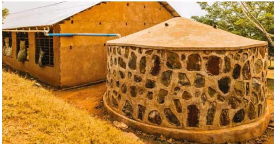
Three new water tanks constructed for primary schools in Kagera
