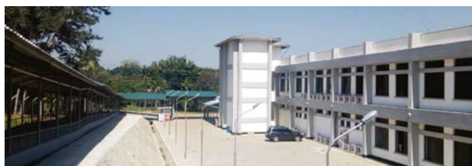
Tumbi Regional Referral Hospital, Expansion Project, Main Building
