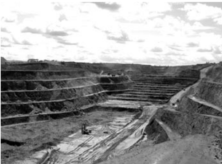
The Golden Pride pit. The mine is owned by Resolute Mining with Moolman Mining (East Africa) acting as the mining contractor. Like most of the mines in Tanzania it is an open-cast operation.
